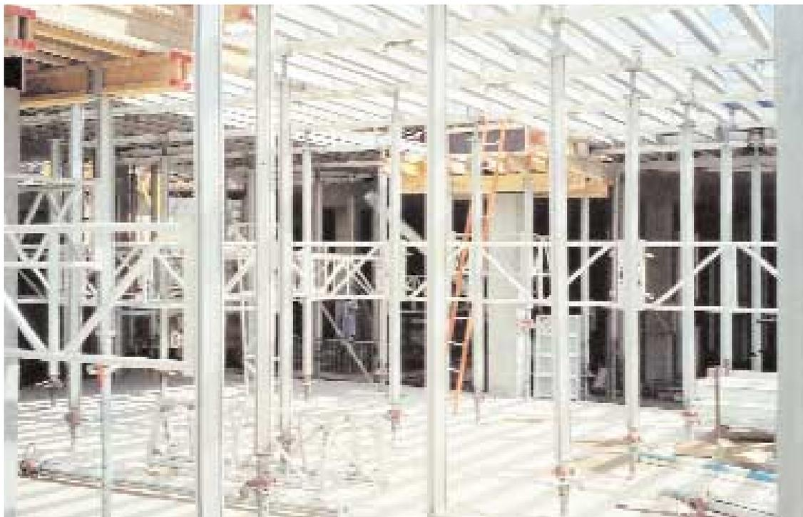
MevaDec slab system in drop head-beam-method.
