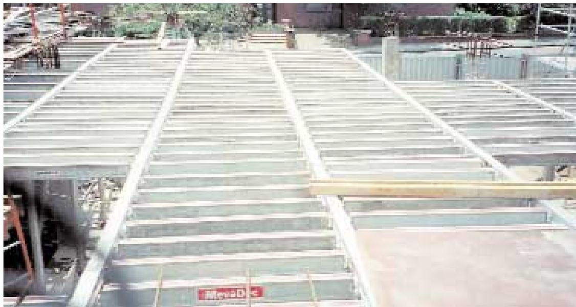
The drop head-beam-method enables the free choice of facing to be placed as a soffit.
